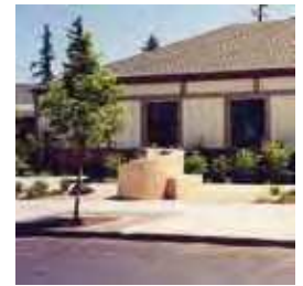
Becky Johnson Community Center
